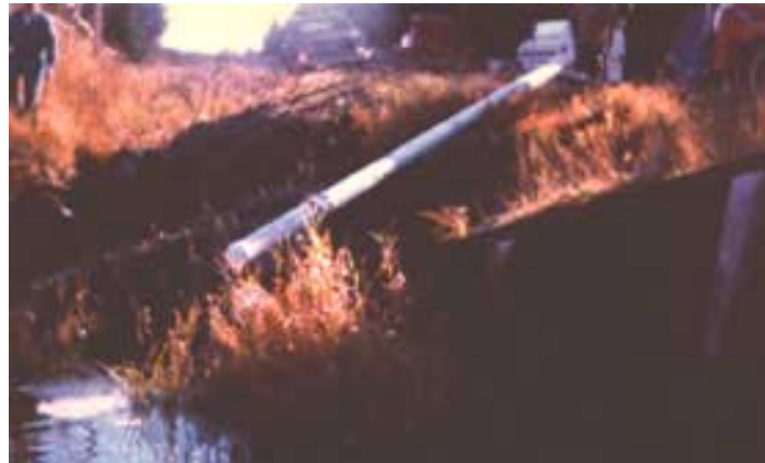
Photo 3: Assembled hydrant system ready for placement in the water.
