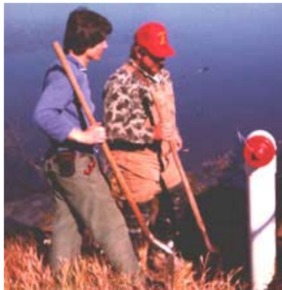
Photo 8: Hydrant connection installed on pipe so that it is below the pump intake.
