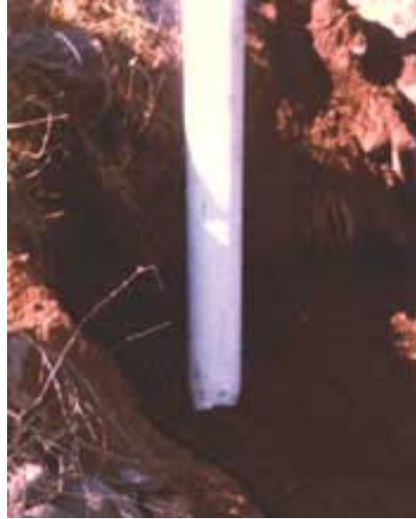
Photo 7: Riser pipe extending above ground before being cut to proper height.
