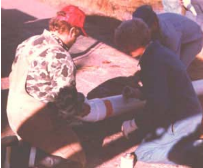
Photo 1: Gluing pipe fittings together and taping joints.
