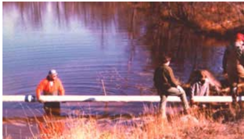
Photo 4: Aligning pipe assembly with the trench.
